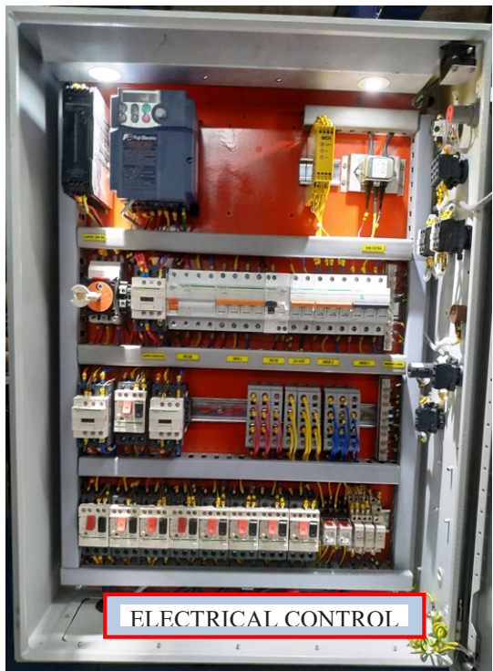
RCCB & MCB SAFETY EQUIPMENTS
